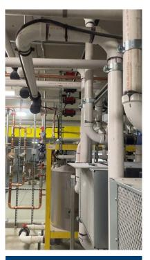
By installing AcornVac's water-saving vacuum plumbing system in its renovation of an historic office building, Holaday-Parks earned the building recognition for environmental sustainability. The building's AcornVac mid-level waste collection tank captures waste from upper-floor fixtures; here, it is supported by a framework.
